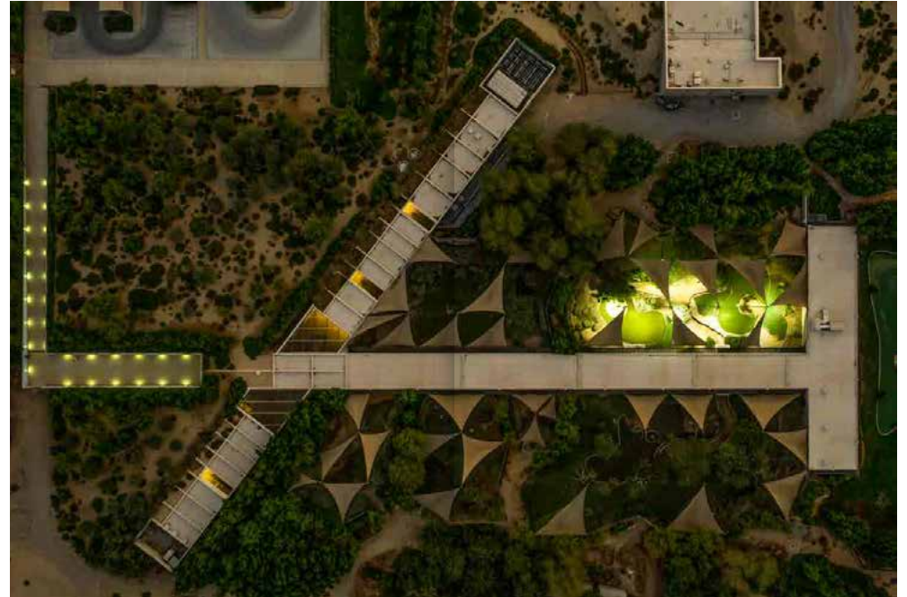
A photograph taken from above soon after completion shows the graphic precision of the architecture, derived from the building as a series of walkways.
