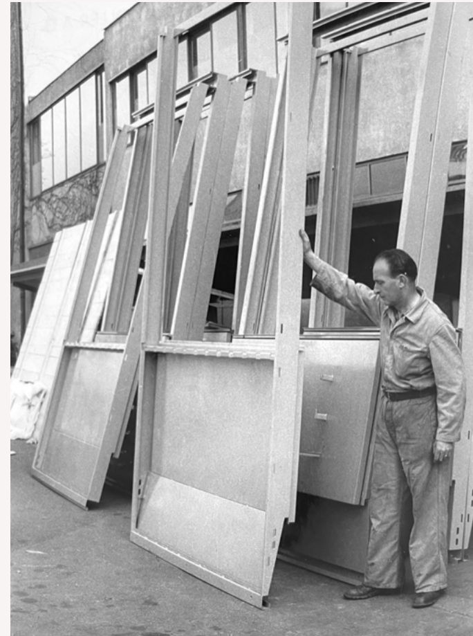
Prefabricated façade elements, Metallbau Koller AG.
