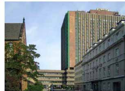
Fig. 1 A twenty-one-story hospital tower was added to the historic Charité complex in 1962.
