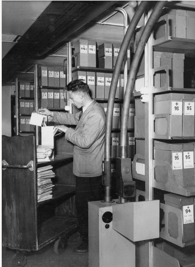
Patent magazine and pneumatic dispatch system. ETH Zurich, main building, ca. 1952.
